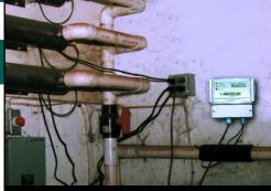
Triangular Wave Deposit Control System treats water before the water enters the UV disinfection units, keeping quartz sleeves clean
