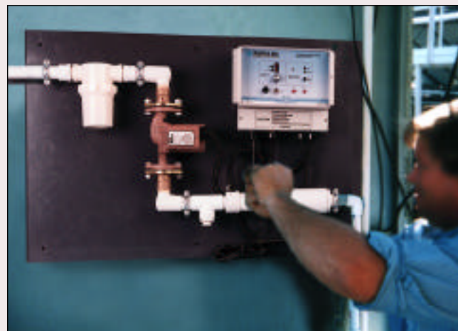
Side Stream ByPass HVAC Treatment System
