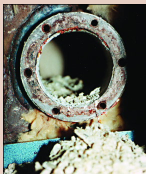
Scaled Hot Water Pipe
