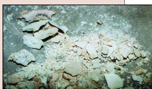
Pounds of Scale Removed from a Hot Water Plumbing and Heating Systems
