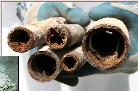
Scale Encrusted Scale Pipes
