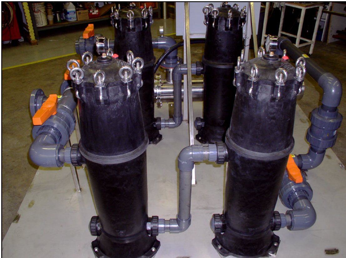
Rear View Staged Filtration
