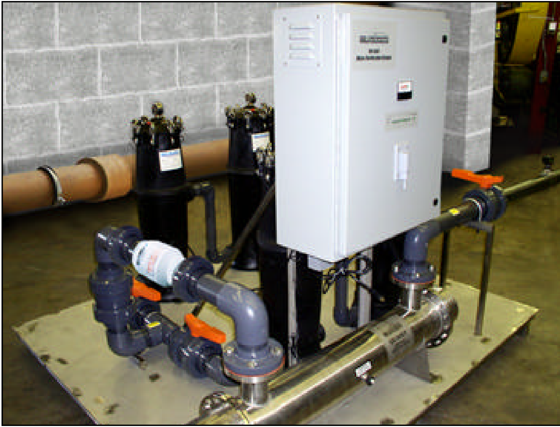
Front View Control Panel
