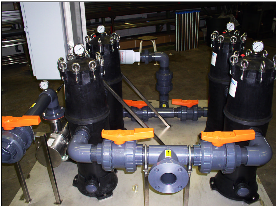
Side View Right 3" Plumbing In/Out of System
