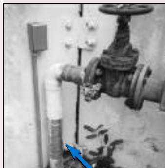
The coil is wrapped around a water pipe and protected from dirt, disturbance and moisture with weatherproof tape.
