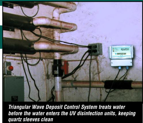
**Triangular Wave Deposit Control System treats water before the water enters the UV disinfection units, keeping quartz sleeves clean**
