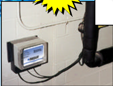
TWT® Deposit Control unit, installed on water feed line point-of-entry for water conditioning at commercial facility.
